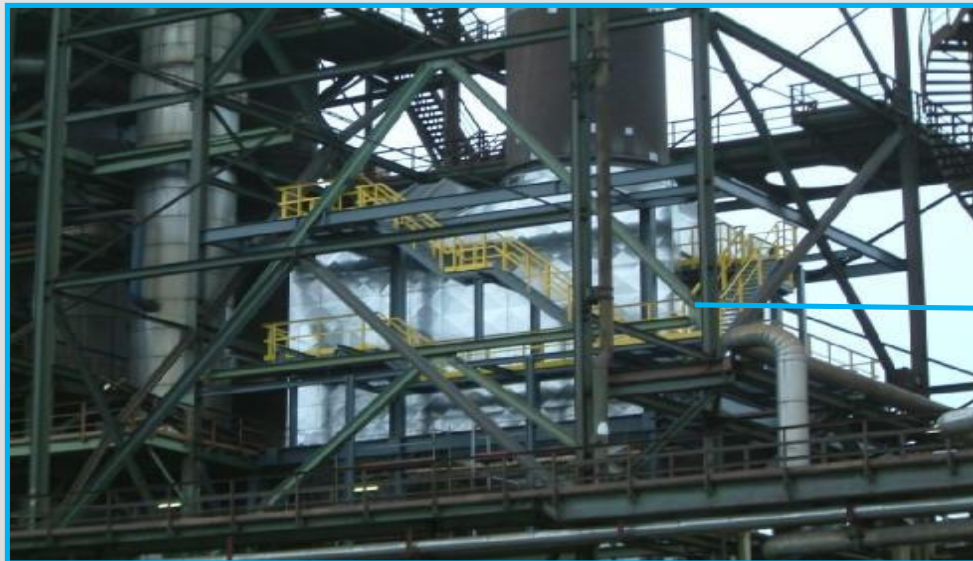
Ecostat-Heat Pipe – Replacement of a different type of heat exchanger at Voest BF, Austria
