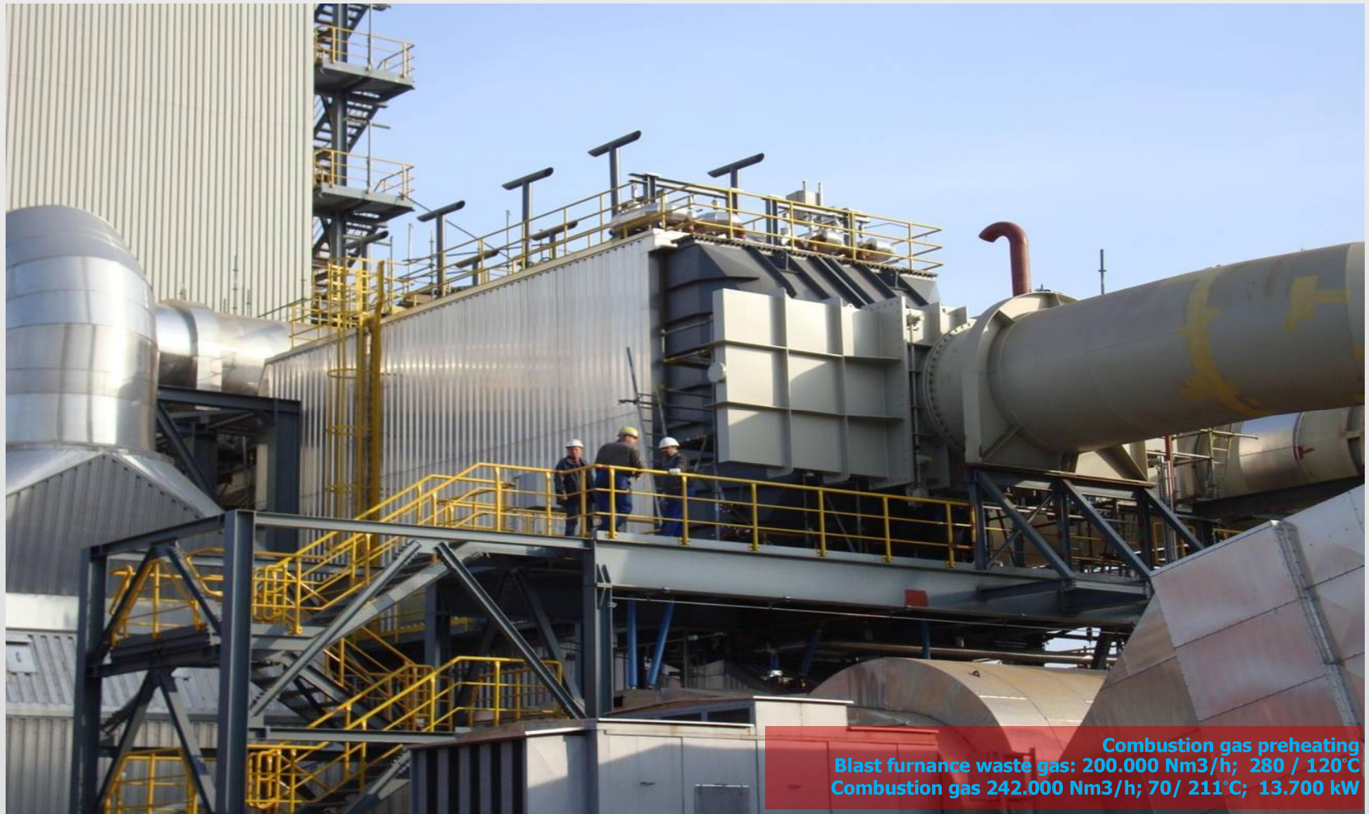
Ecostat-Heat-Pipe-System - GKW Dillingen (blast furnace gas power plant) – real execution -
