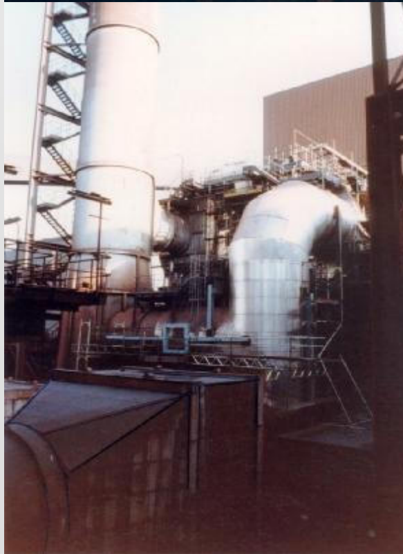
Ecoflow in steel industry waste heat recovery from sinter cooler at TKS Duisburg Schwelgern for air and gas preheating at BF1
