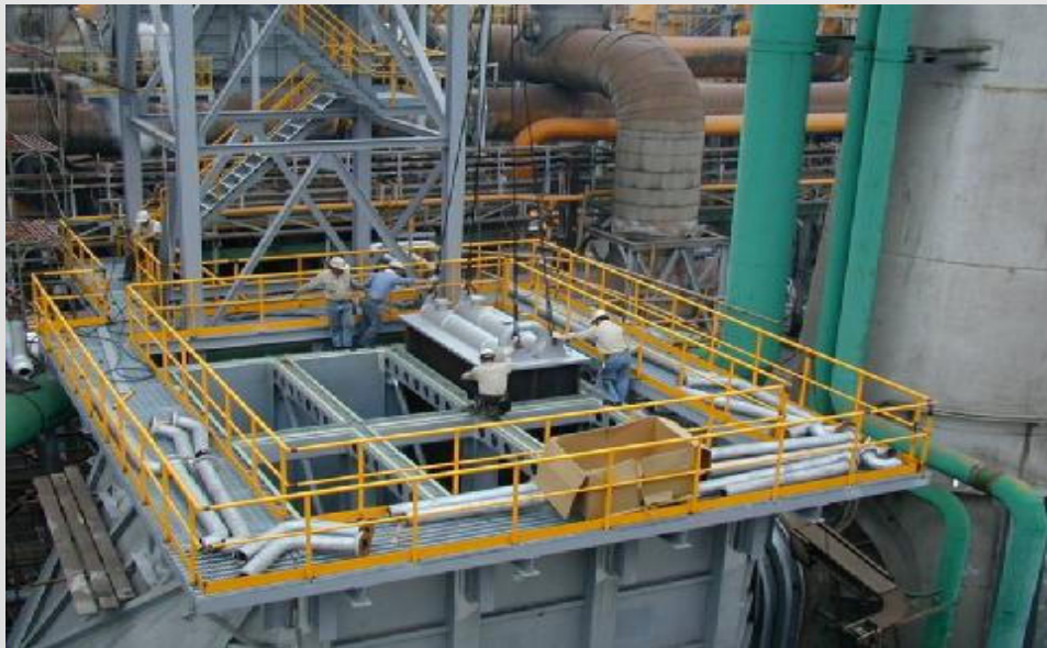
Ecoflow with thermal oil in steel industry, erection at CSC Taiwan BF3 waste gas side heat exchanger
