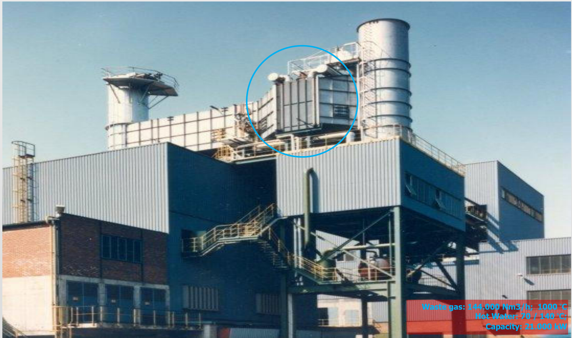
Ecoflow in steel industry waste heat recovery from cupola furnance at Eisenwerk Brühl to gernerate hot water via thermal oil
